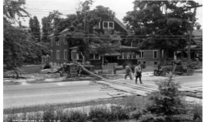
Chenango St, still brick, near Terry Ave, after the 1935 flood.
